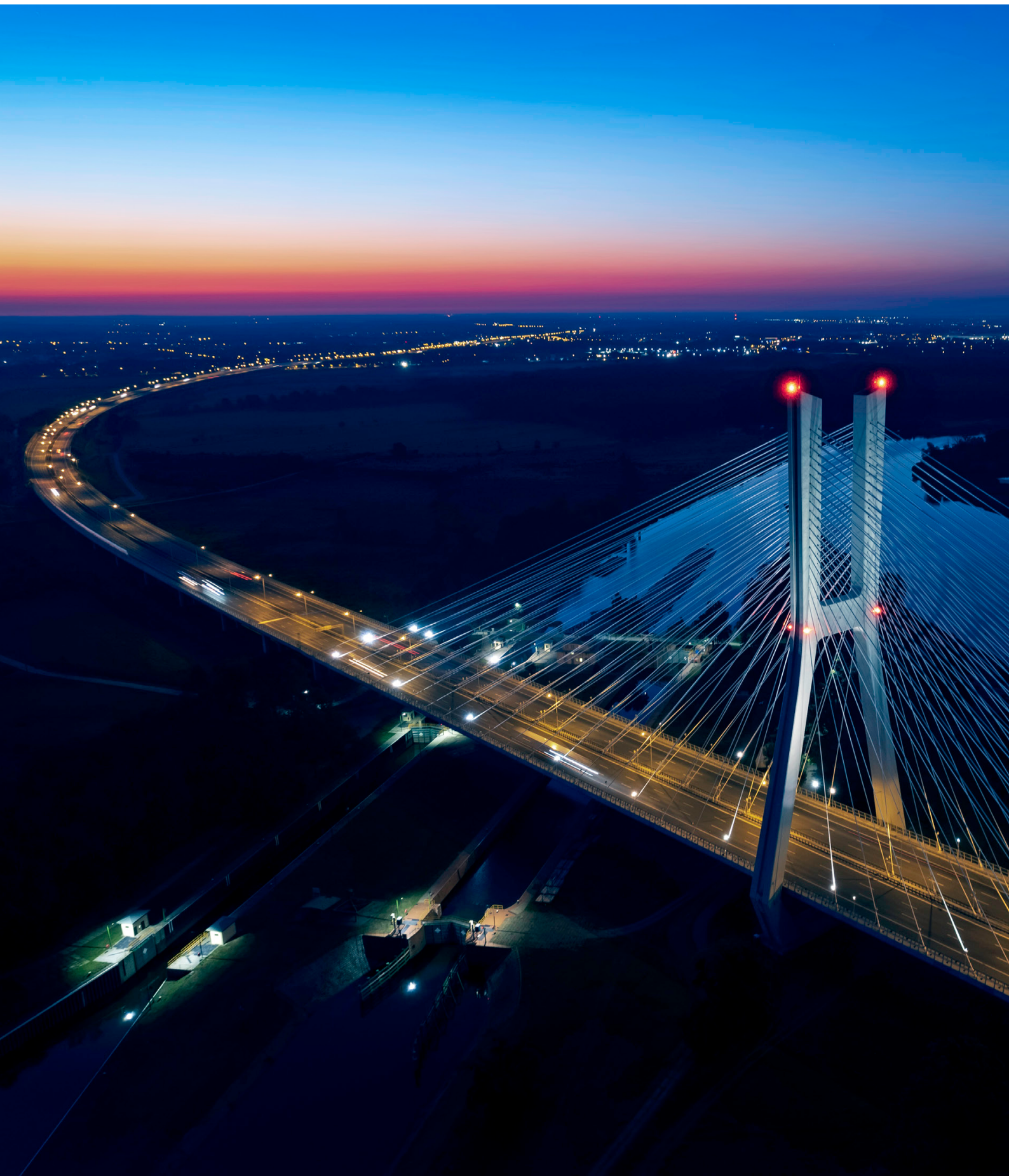
Bridge over the Odra river in Wrocław, Poland © Adam Smigielski/Getty Images
