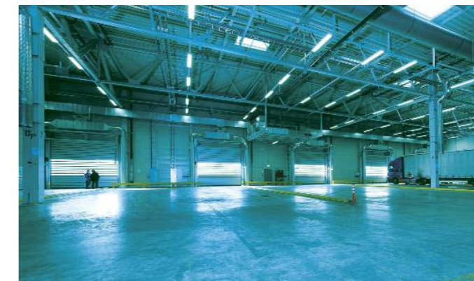
Green logistics: Warehouse tenants are increasingly demanding that landlords implement sustainable solutions that would enable them to offset their environmental footprint.
